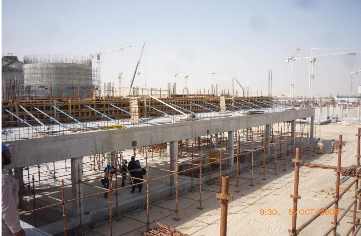
W104- Workshop Building
