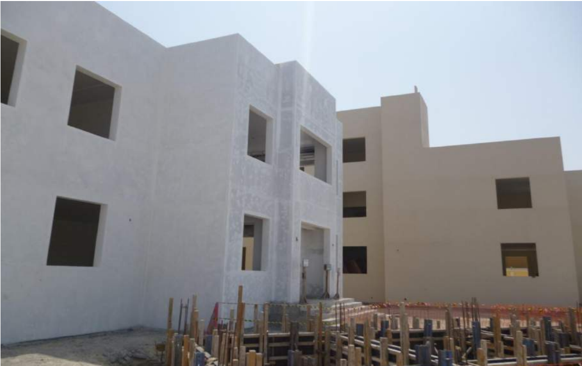
External Finishing Work
