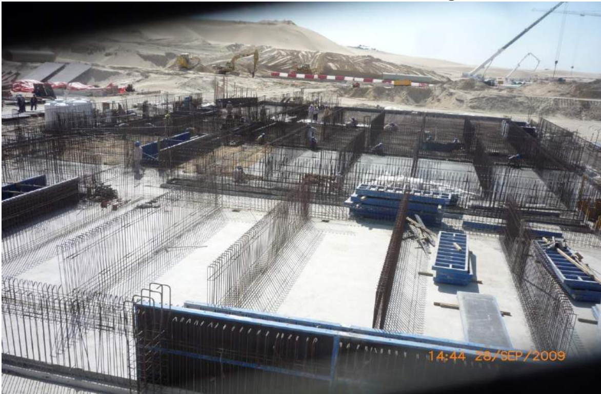
W30-Disc Filter Building
