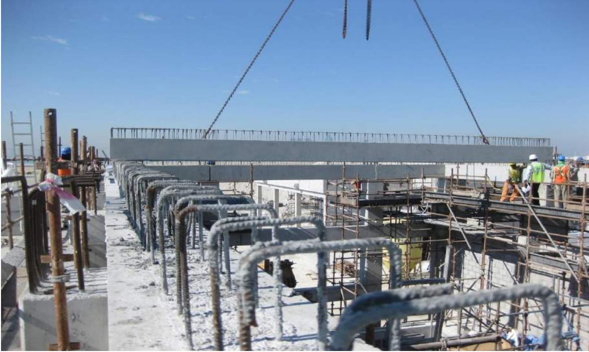
Precast Beams – Pre-Treatment Building
