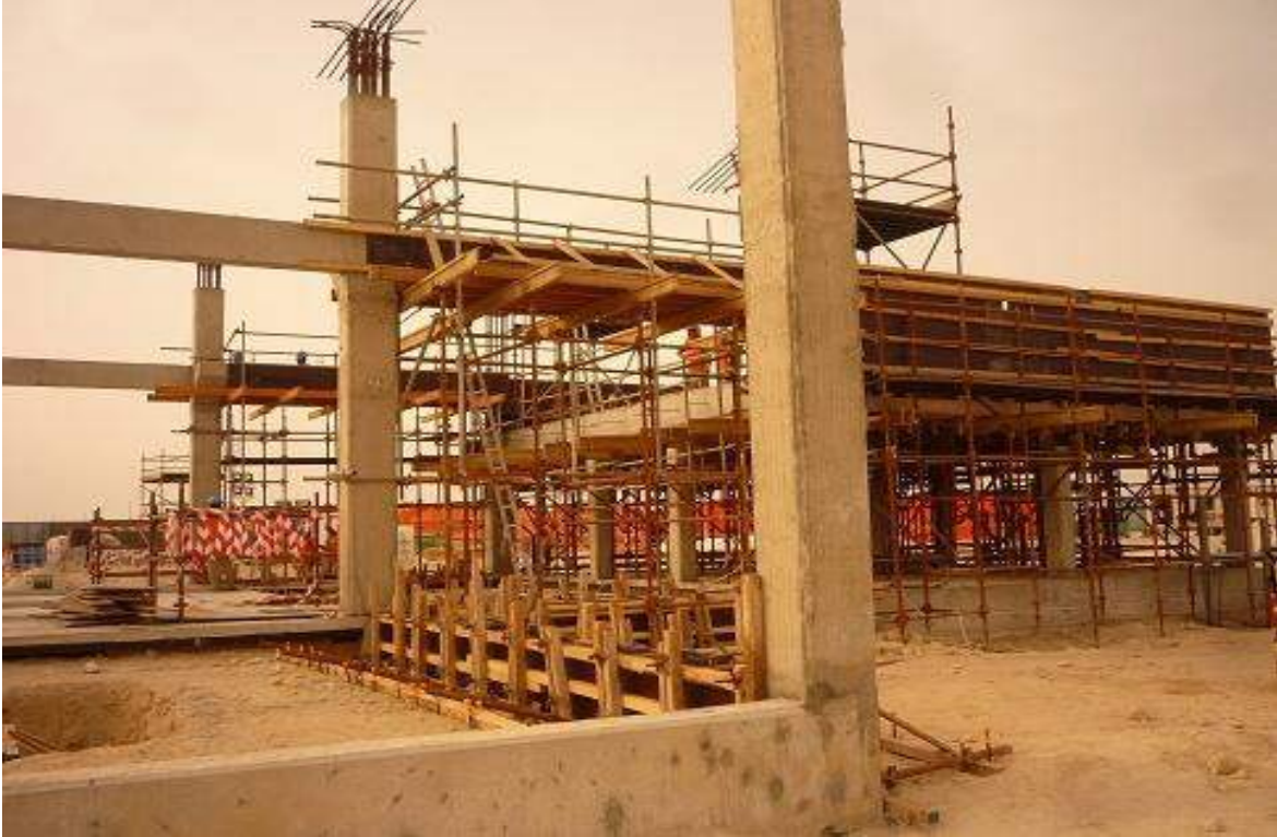
Sludge Dewatering Building
