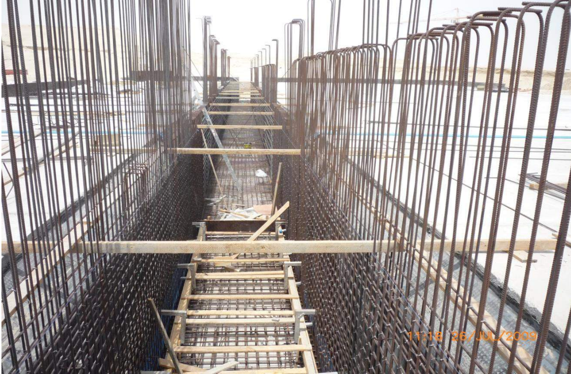
Trench Wall @ W30-Disc Filter Building
