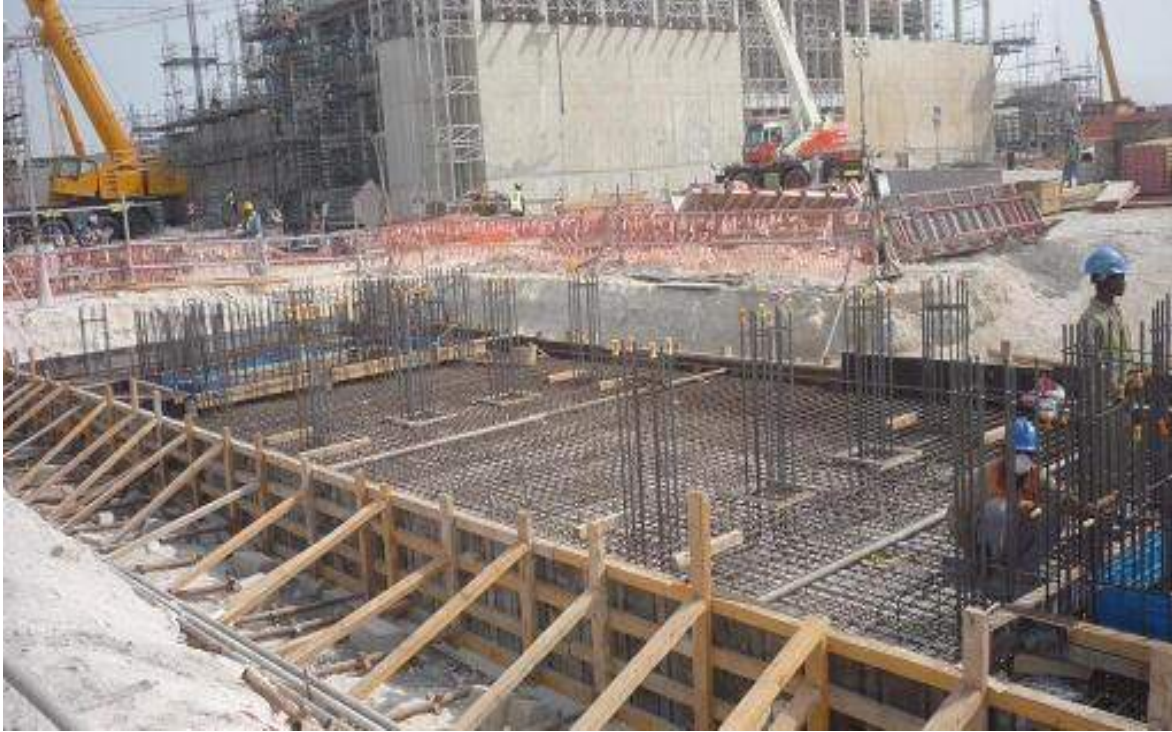
UV Channels & Disinfection Building
