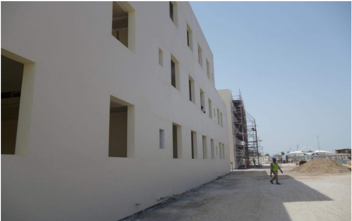
External Painting Works
