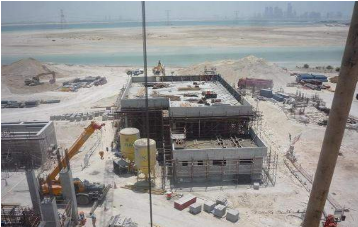
Sludge Dewatering Building
